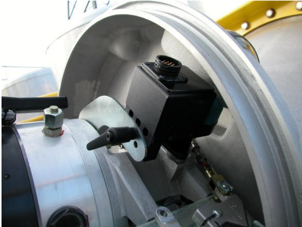
Rotary Transducer on ABB HMB Mechanism
